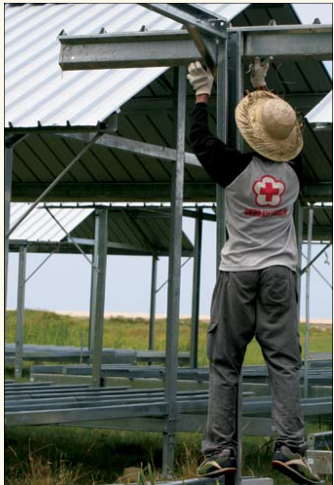
An Indonesian Red Cross worker constructs a steel-framed, transitional shelter.
